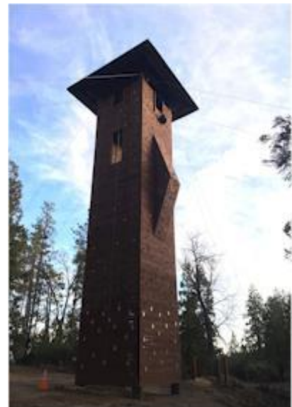
NEW 60 foot climbing tower Tallest tower in the Boy Scouts of America!
